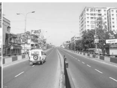
Gariahat Flyover, Calcutta at 10-30 a.m.
